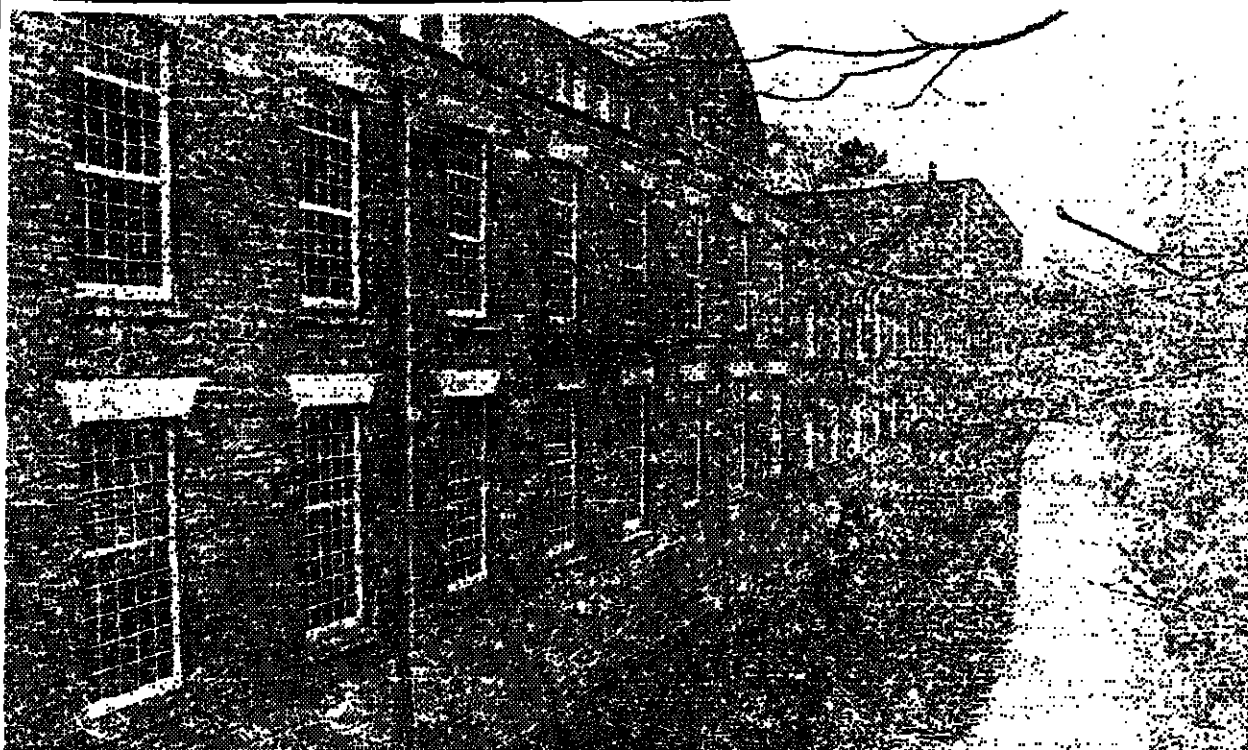
King cotton: Quarry Bank Mill, founded in 1784 by Samuel Greg. His workers' quarters were above the usual standard
